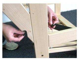
Insert the threaded ends into the holes through the uprights and warp beam supports, slide on the washers and fasten the wing nuts.
